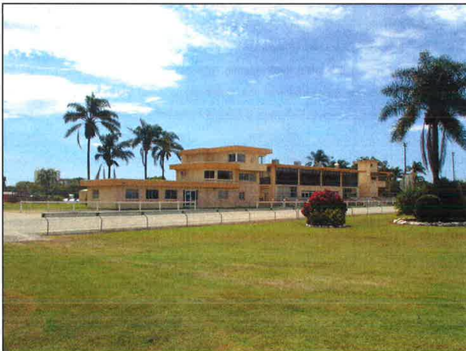
Figure 25: View north east to the racing complex and betting auditorium of Border Park Raceway
